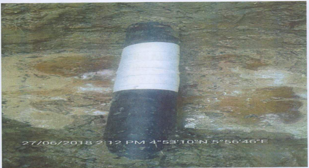
HACKSAW CUT ON THE FACILITY.
