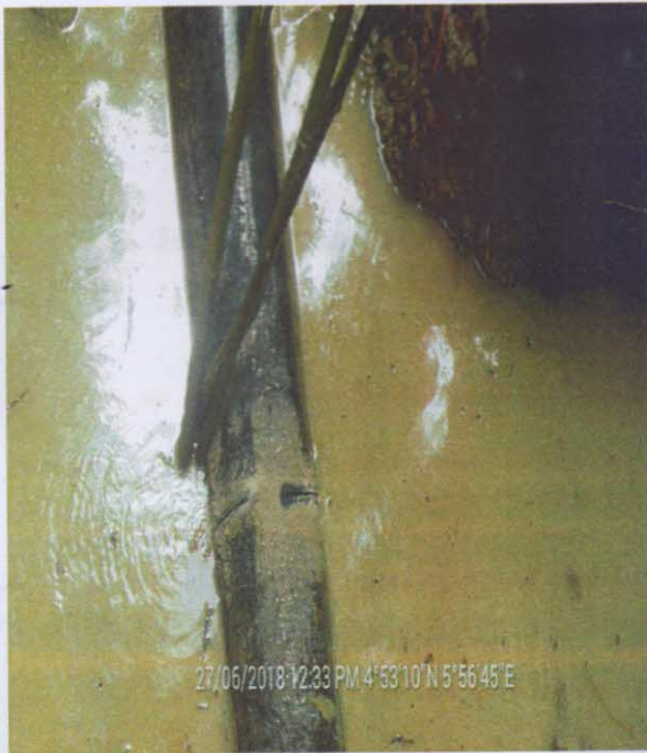
HACKSAW CUT ON THE FACILITY.
